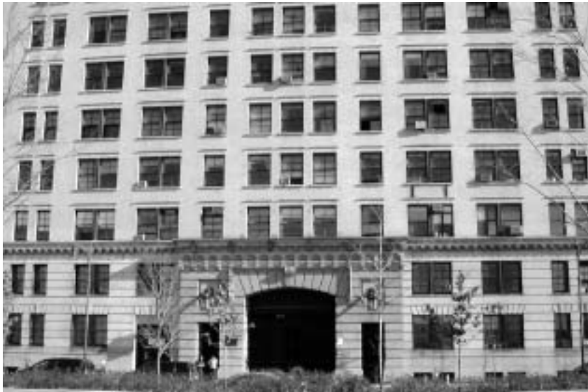
Fig. 15. Westbeth, 463 West Street. Photograph by the author.
